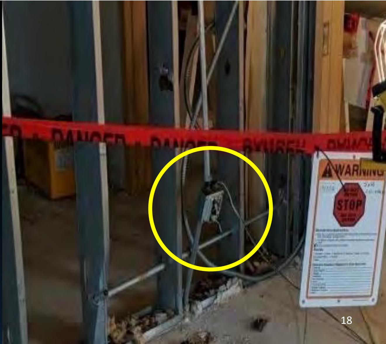
Snippets used by the construction worker were not insulated. The arc blew one tip off and left a half moon on the other side.
